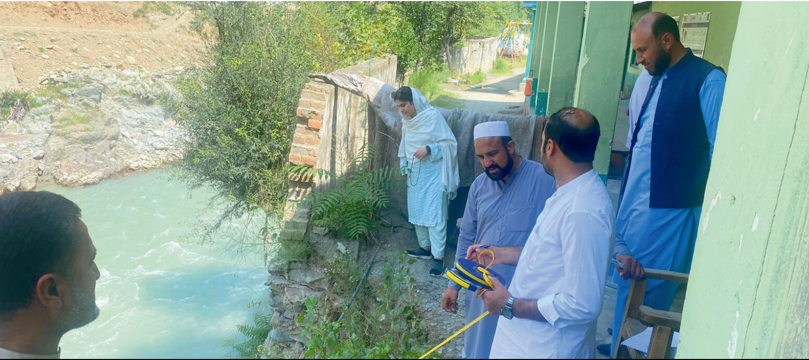
ISU-DoE&SE, along with PTC and teachers, inspecting the damages at a flood affected school
