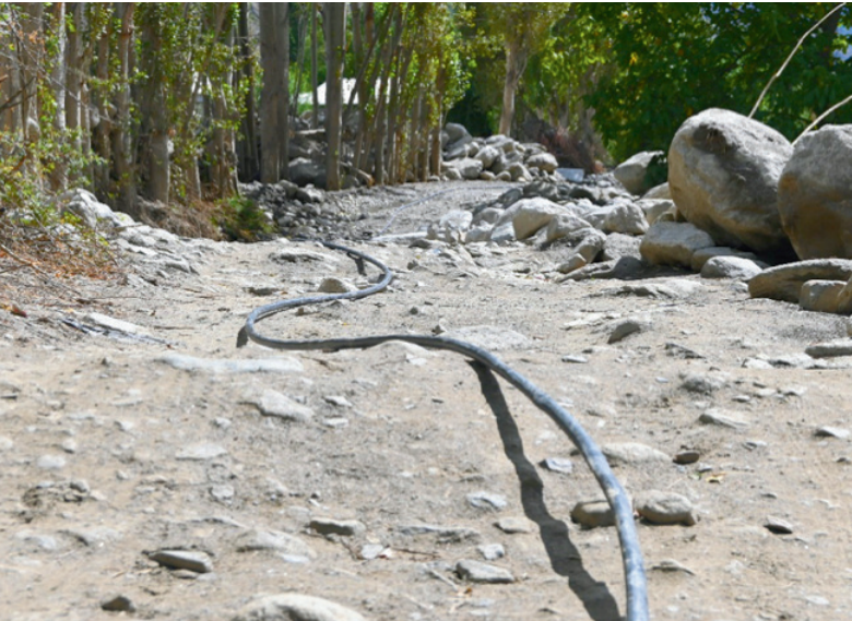
Installation of a 355-foot water pipeline, ensuring clean water supply from the designated water source to school
