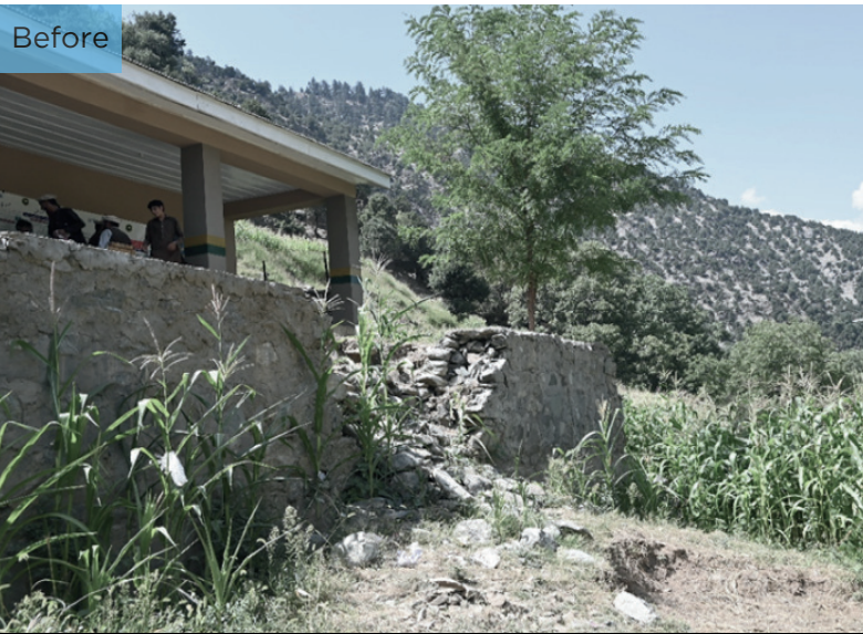
(LEFT) Damaged retention wall (RIGHT) Rehabilitation of the retention wall with fencing for additional safety
