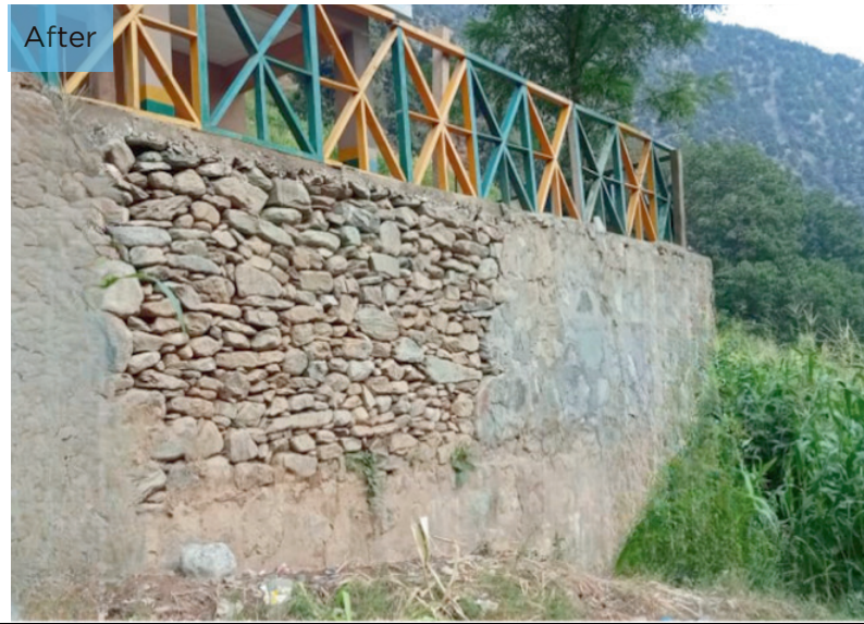
(LEFT) Damaged retention wall (RIGHT) Rehabilitation of the retention wall with fencing for additional safety
